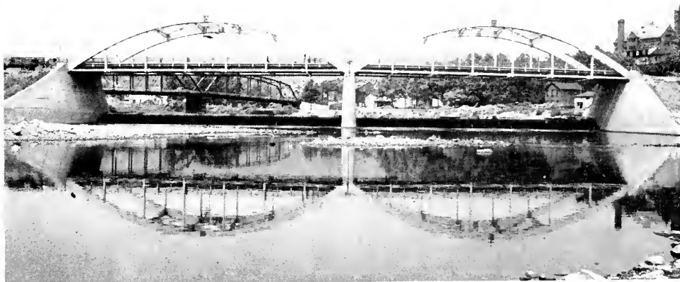
Cumberland's new Blue Bridge.
